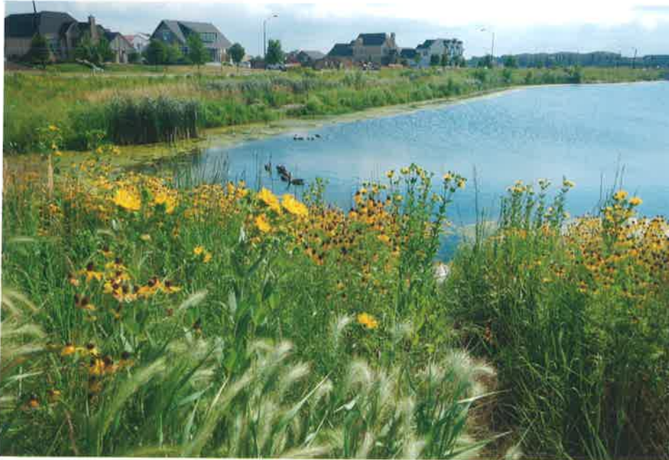
This pond is part of a series of natural treatment areas for stormwater. It was designed using the unified sizing criteria and it creates an open, park-like setting for residents to enjoy.
