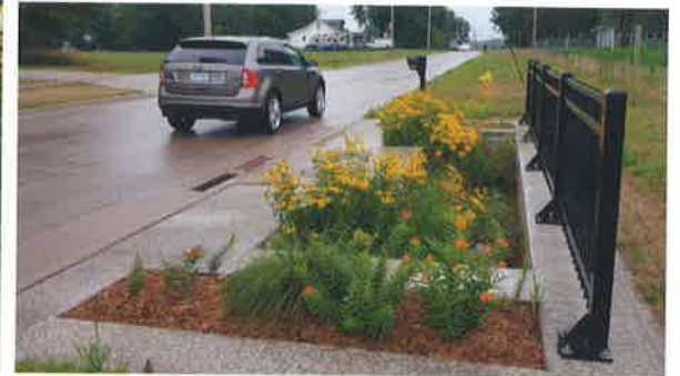
Permeable pavers (top) and bioretention cells (bottom) also soak in rainfall and manage stormwater where it falls instead of shedding polluted water.
