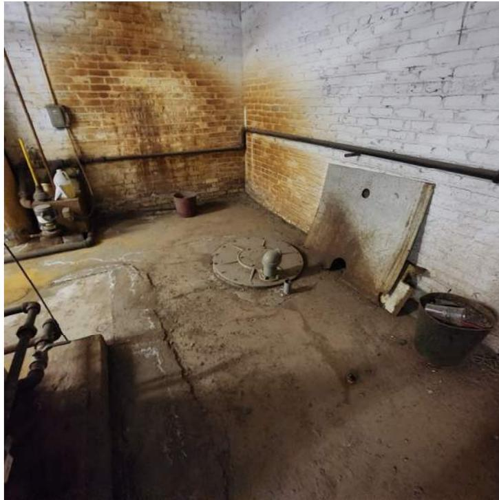
**Photo 17** – Potential fuel oil tank (previous Phase I ESA provided by property owner noted it was filled in place).
