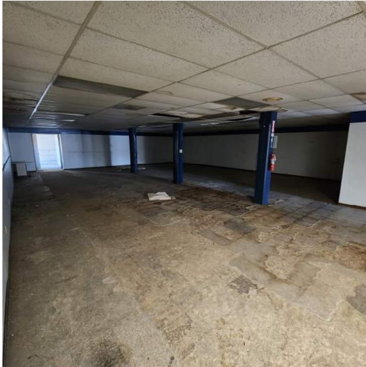
**Photo 8** – 1<sup>st</sup> floor office area with dampness/mildew smell and water damage.
