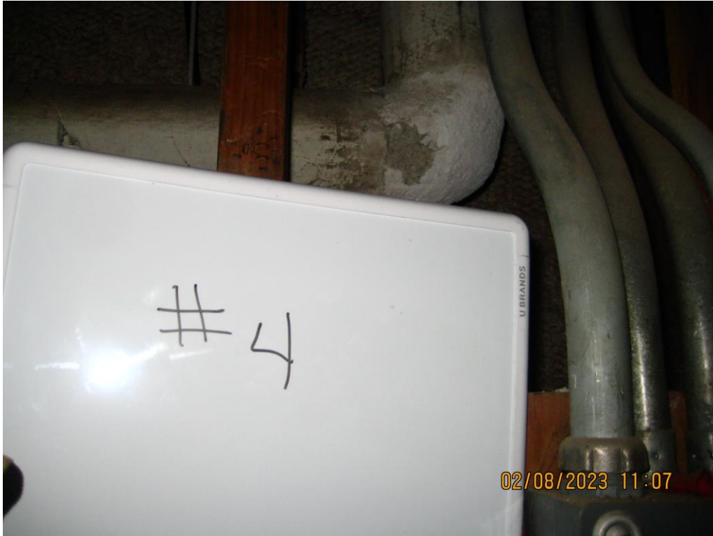
Sample #4 – Pipe Fitting (SE Basement Stairwell)
