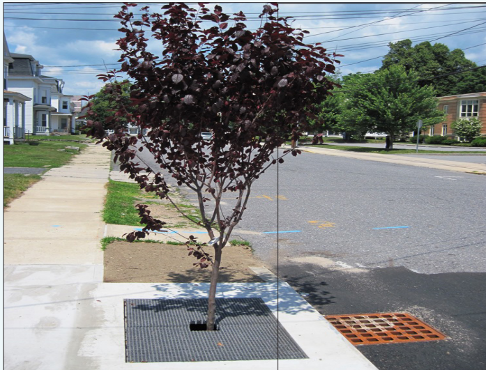
Stormwater Tree Filters, an “in-street” practice integrated into the storm drain inlet and a last line of defense to runoff control.
