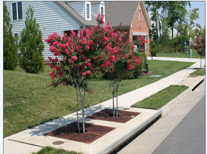
Stormwater Tree Filters, an “in-street” practice integrated into the storm drain inlet and a last line of defense to runoff control.
