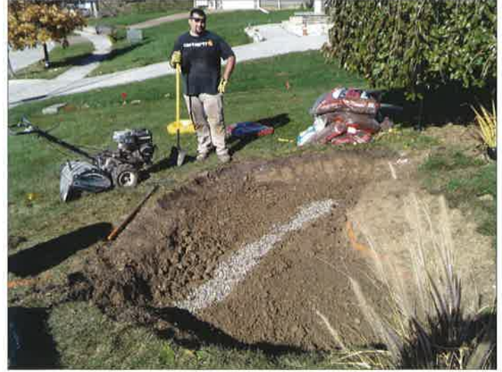
Step 2 Excavate existing soil
