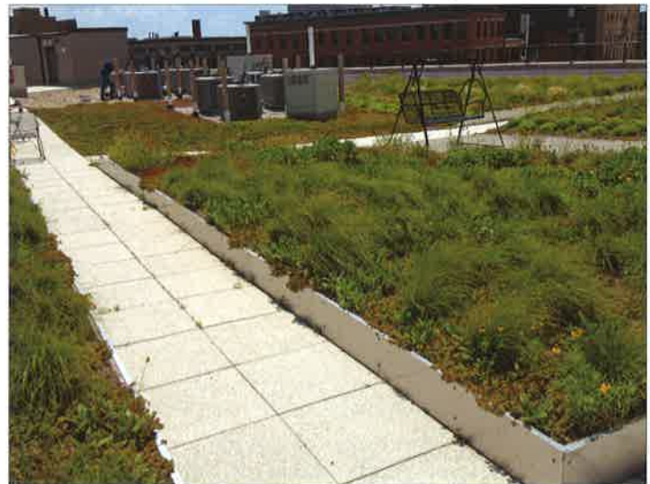
Quad Cities semi intensive rooftop has soil depths ranging from 4-8 inches.
