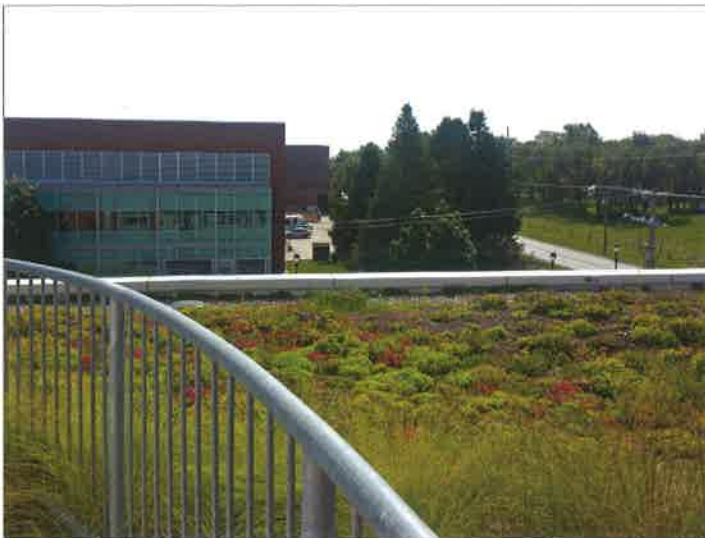
Semi intensive green roof at Central College in Pella supports more plant diversity.
