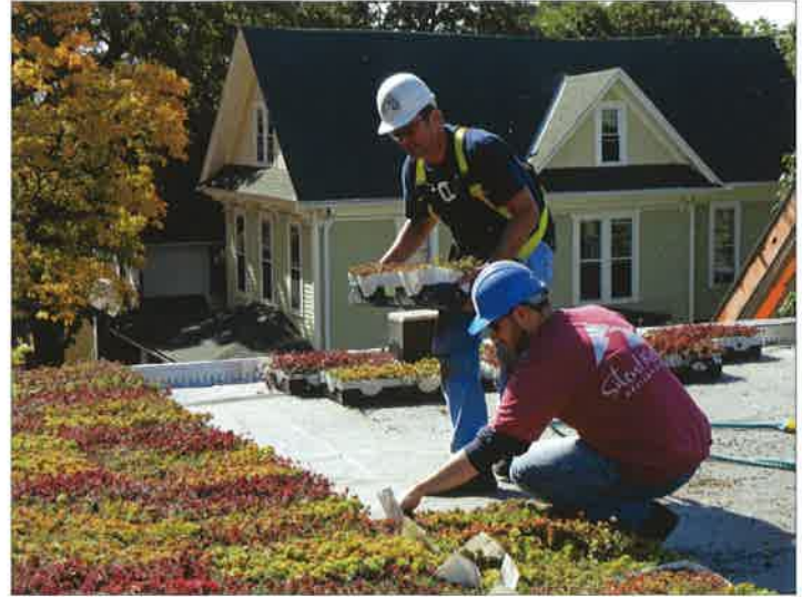
Sedum tray system is installed in Des Moines.
