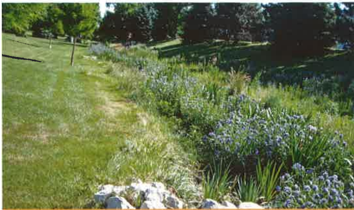
This Davenport bioswale is solving the problem shown in Picture 1 on the previous page. A wet, eroding neighborhood drainageway is now an attractive and functional stormwater system with native grasses and flowers.
