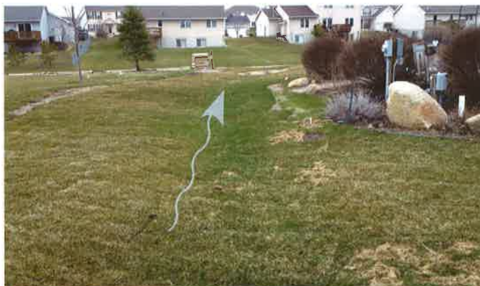
Most people would not realize that a stormwater practice is installed at this site. This Cedar Falls backyard bioswale will ensure a dry, mowable, and usable water management area. Permeable soil, a perforated subdrain and subtle earthen berms help infiltrate most runoff. Mow turf grass as high as possible to maximize vegetative cover.
