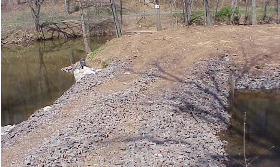
Figure 4.4. Temporary stream crossing (Source: F. X. Browne, Inc.)
