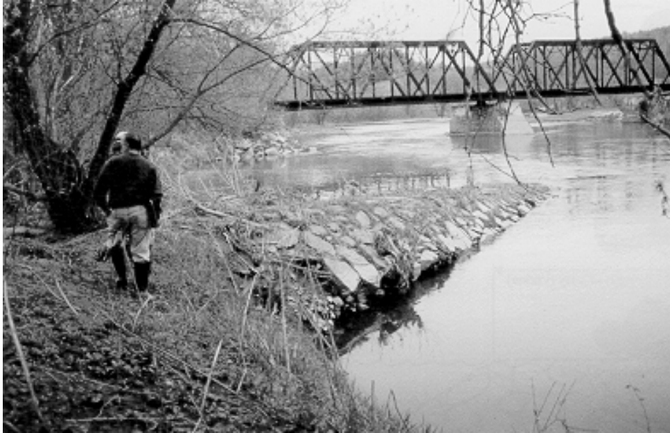
Figure 3.21. Jetty (Source: Department of Civil, Construction, and Environmental Engineering, Iowa State University)
