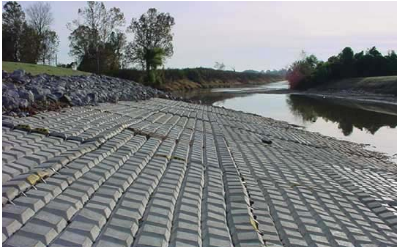
Figure 3.31. Streambank protection (Source: International Erosion Control Association)
