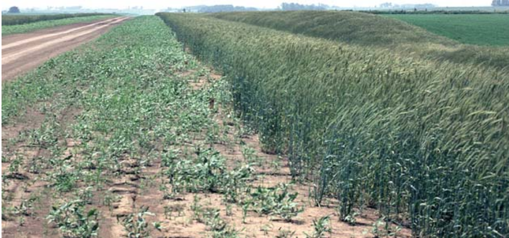
Figure 2.20. Roadway filter strip (Source: Iowa DOT)
