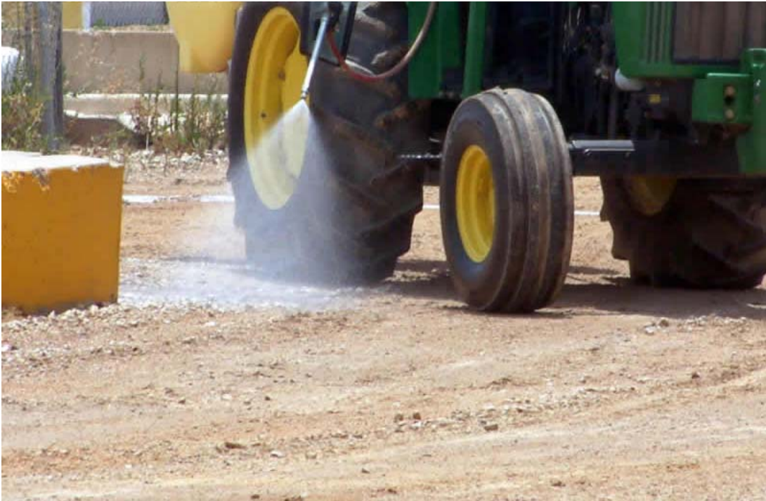
Figure 2.6. Manual dust-control applicator (Source: http://soiltac.com/Photo_Gallery.html )
