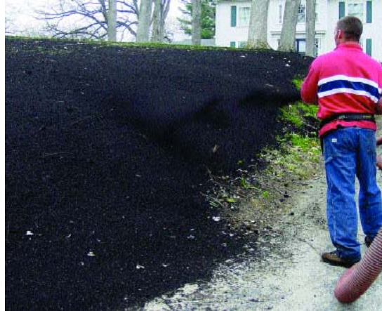
Figure 2.23. Blown compost blanket (Source: Iowa Natural Resources Conservation Service 2004)
