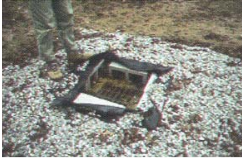
Figure 3.14. Inlet protection (Source: Minnesota DOT)
