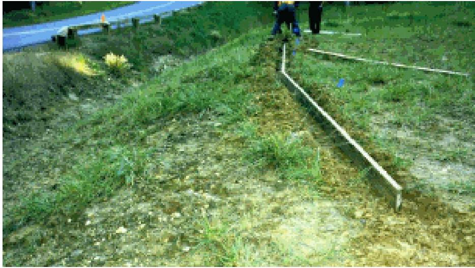
Figure 3.23. Level spreader installation (Source: William B. Umstead State Park)
