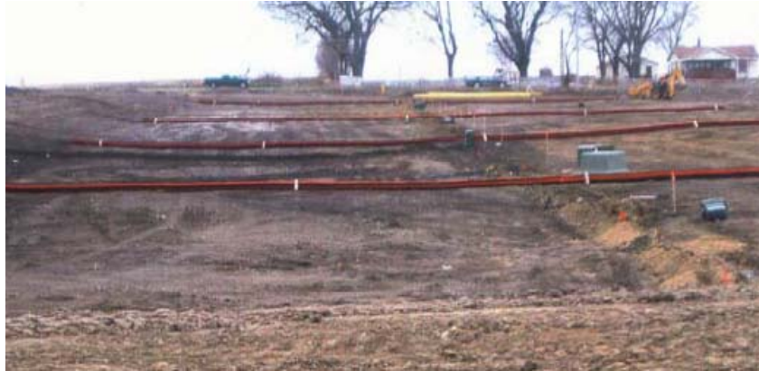
Figure 2.24. Compost filter tube (Source: SUDAS Design Manual)
