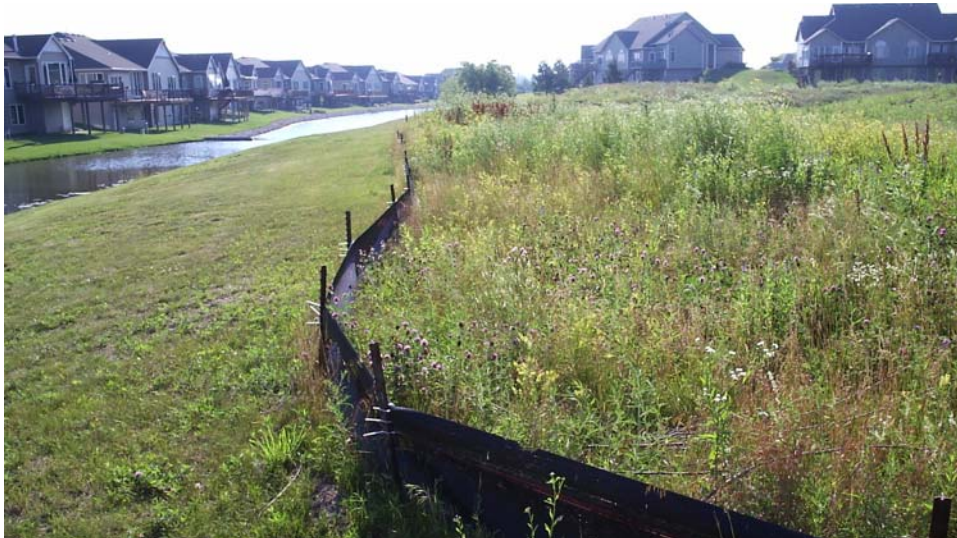
Figure 2.22. Urban filter strip (Source: Department of Civil, Construction, and Environmental Engineering, Iowa State University)
