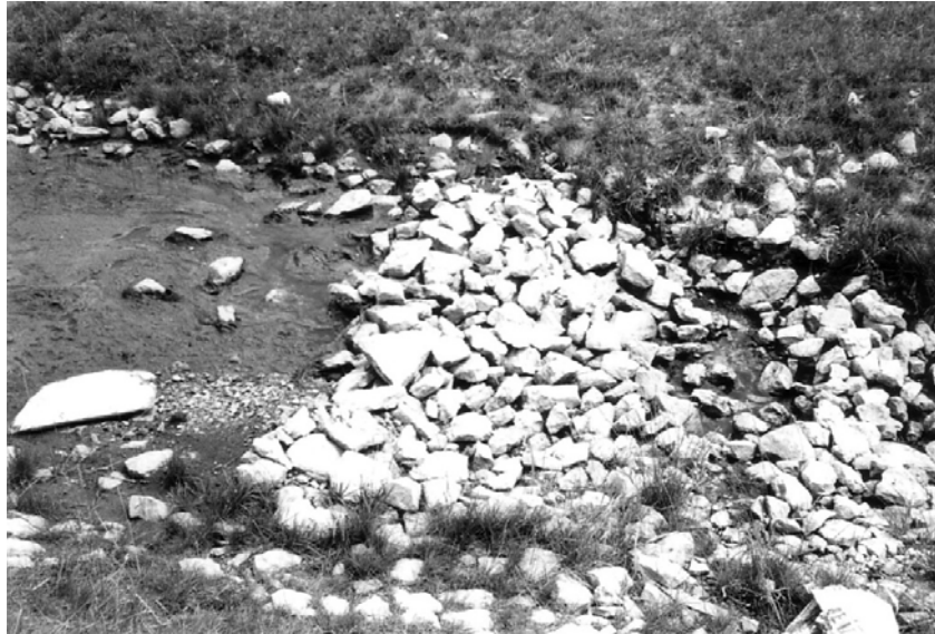
Figure 3.7. Check Dam (Source: Department of Civil, Construction, and Environmental Engineering, Iowa State University)
