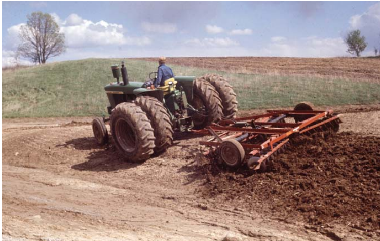
Figure 2.19. Surface roughening by disking (Source: Iowa DOT)
