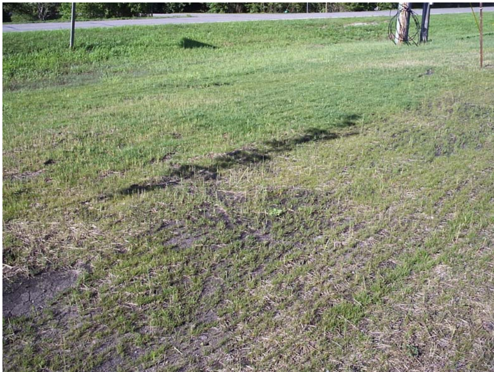
Figure 2.9. Grain drill seeding (Source: Department of Civil, Construction, and Environmental Engineering, Iowa State University)
