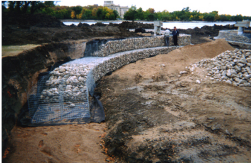
Figure 3.13. Gabion (Source: Modular Gabion Designs)
