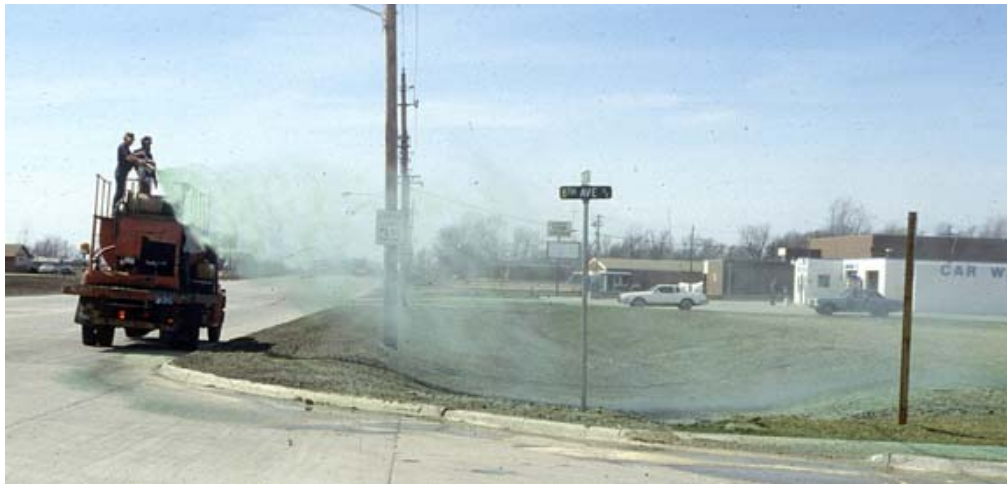
Figure 2.8. Seeding and fertilizing (Source: Iowa DOT)
