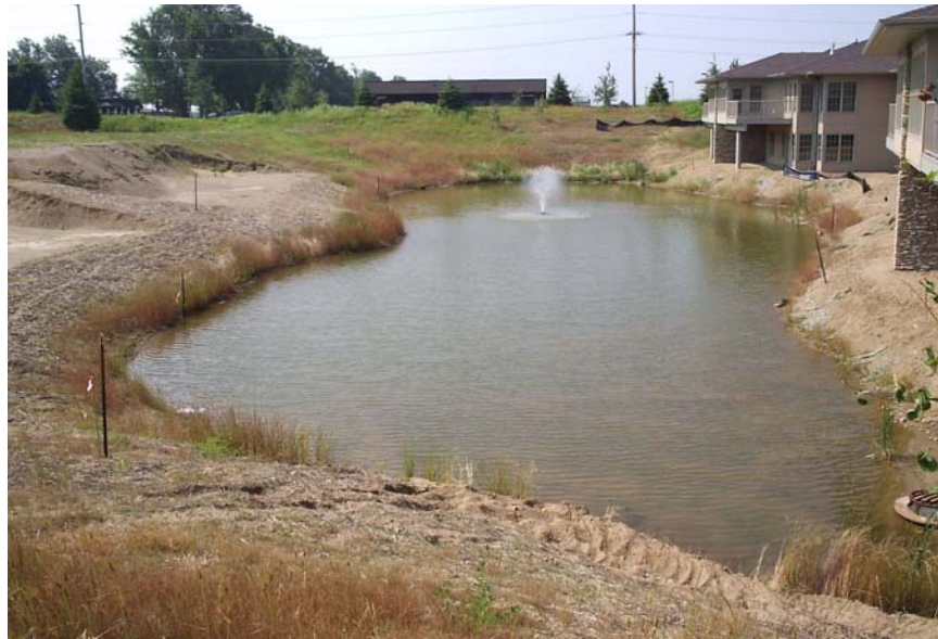
Figure 4.2. Retention pond (Source: Department of Civil, Construction, and Environmental Engineering, Iowa State University)
