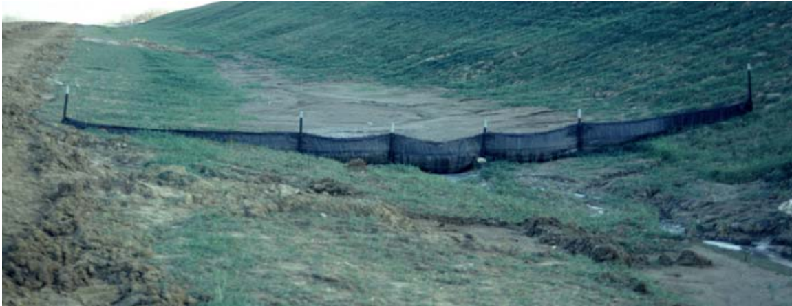
Figure 2.10. Silt fence (Source: Iowa DOT)
