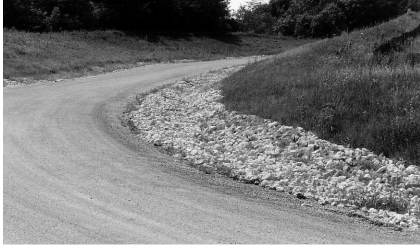
Figure 3.27. Riprap (Source: Department of Civil, Construction, and Environmental Engineering, Iowa State University)
