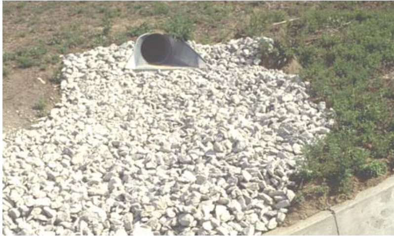
Figure 3.24. Rock outlet protection (Source: Iowa DOT)
