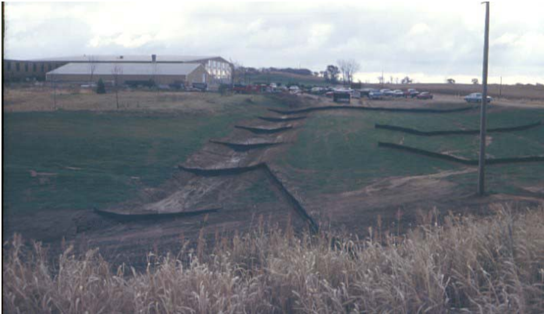
Figure 2.14. Proper silt fence installations (Source: Iowa DOT)
