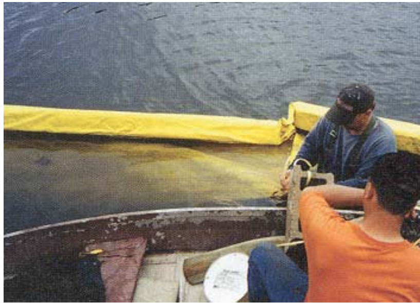
Figure 3.11. Flotation silt curtain (Source: Minnesota DOT)
